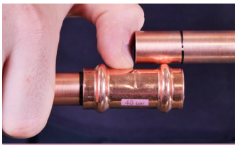
7B. Check the depth mark
